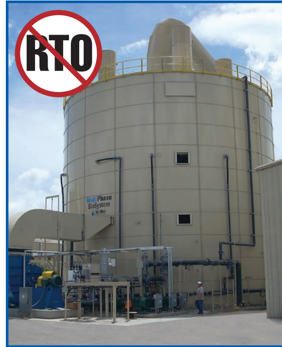
Systems range from 30,000 acfm to 400,000 acfm (300,000 acfm pictured above).
